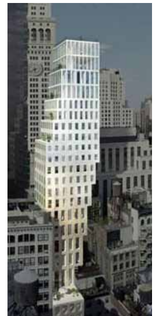
ONE Madison park OMA, app. in aanbouw. E23rd St East Village
