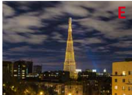
E 1922: Sjabolova tower-zendmast van arch. Shukhov; 160m. adres: Ulitsa Shukhova 8. Metro: Shabolovskaya.
